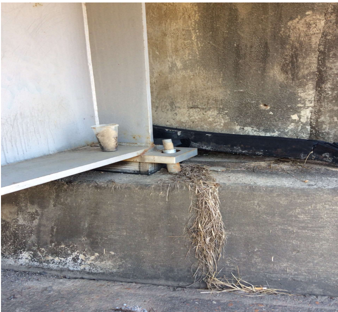
PHOTO 1 Description Anchor Nut missing @ Girder 5 @ Abutment 2.
