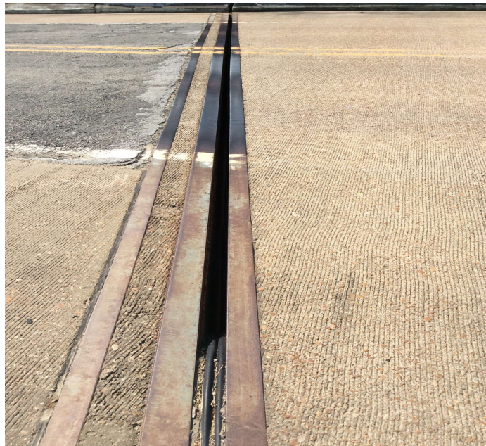
PHOTO 1 Description Abutment 1 - 37' of Joint Seal failed & debris buildup on Cap.
