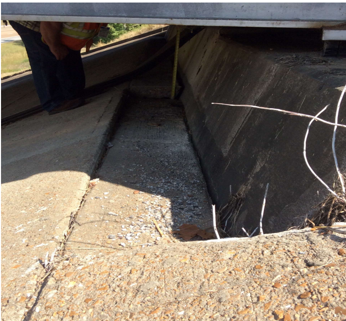
PHOTO 1 Description Concrete Rip Rap settled 4 1/2" @ Left side of Abutment 1.
