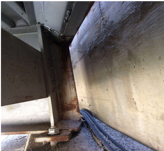
PHOTO 1 Description Abutment 2 has corrosion to bottom of Road Irons & to ends of Girders.
