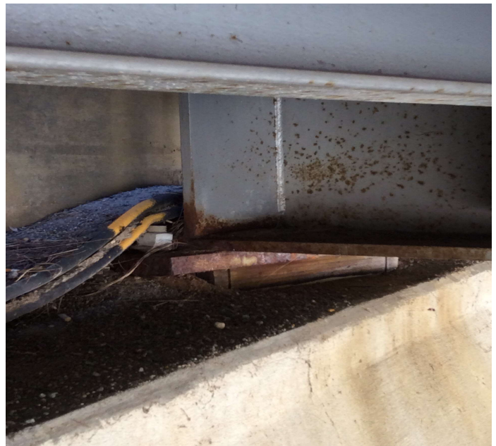
PHOTO 2 Description Typical corrosion to bottom of Road Irons & to ends of Girders @ Abutment 1 & 2.
