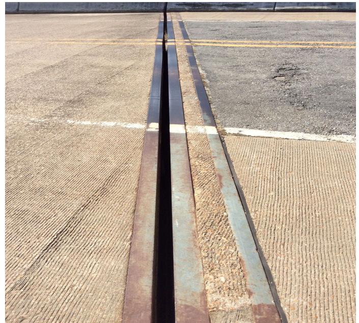
PHOTO 2 Description Abutment 2 - 44' of Joint Seal failed & debris buildup on Cap.
